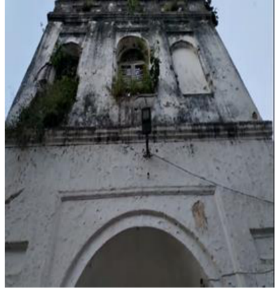
Figure 6 a) Plant growth at the edges of roofs and parapet Figure 6 a) Plants and algae attack
