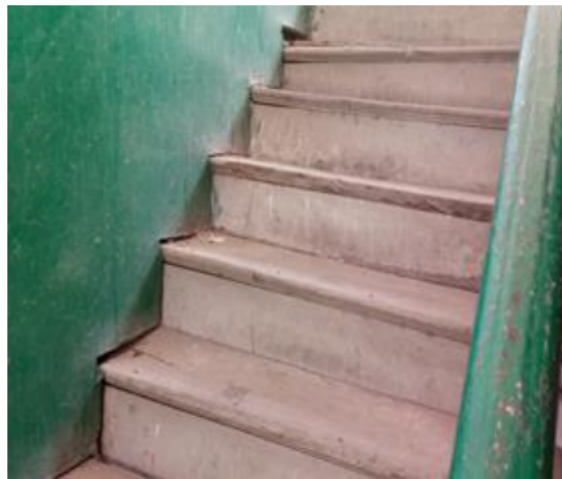
Figure 5 d) Damage in Stair at Circuit House
