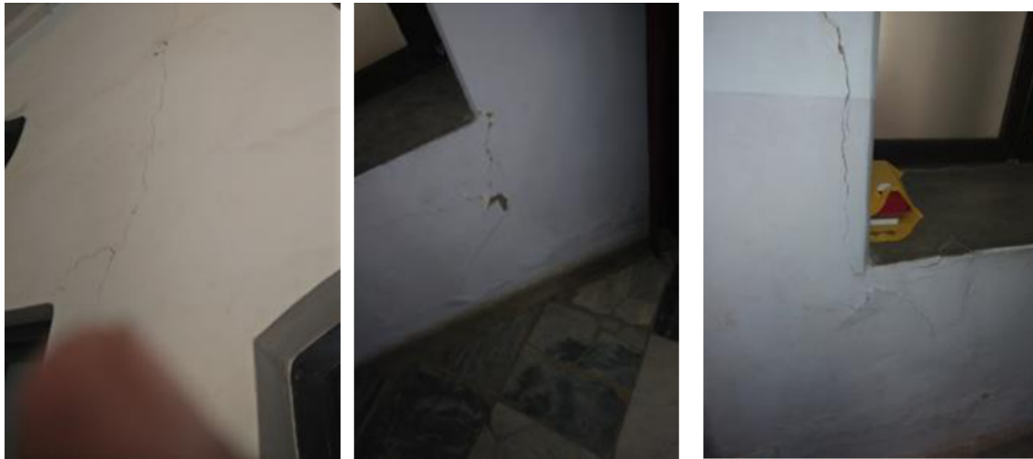
Figure 4 a) Hair line Crack Figure 4 b) Crack due to Settlement Figure 4 c) Structural Crack
