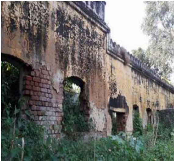
Figure 3 a) Damages to External walls
