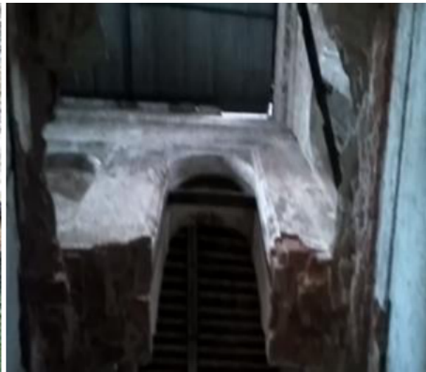
Figure 3 b) Roof and internal wall Damage
