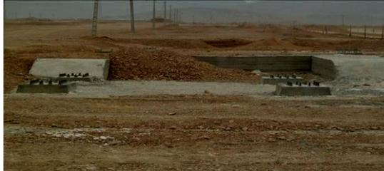
**Figure 4 – A two-levels foundation**
