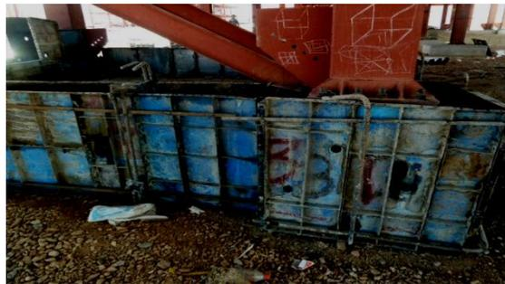
**Figure 5a-Special concrete wall around the lift foundation**
