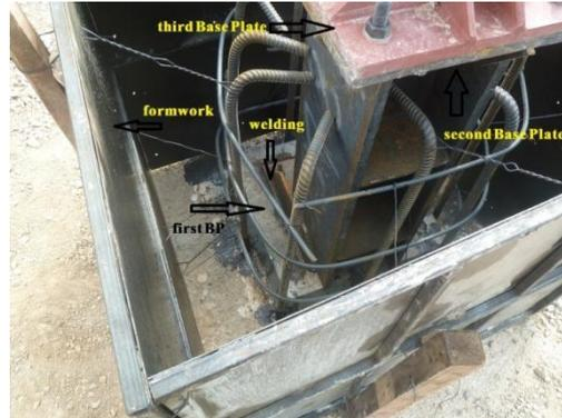
**Figure7 – A pedestal before pouring concrete**
