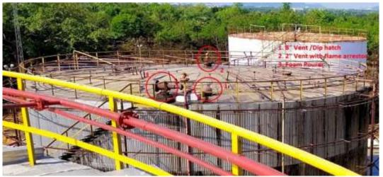
Fig 1: M6 Tank with vents on top of the tank
