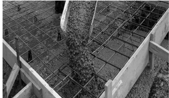
Fig. Geopolymer Concrete in Reinforcement
