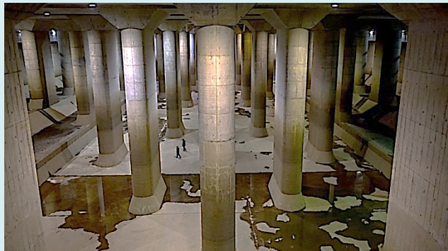
Figure 4: Tokyo underground drainage system - water pressure control bath. (size 178x77x18 meters)
