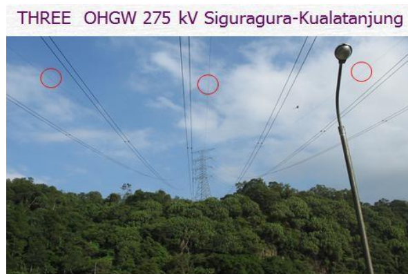
Figure 5. Three earth wire to reduce lightning peak current flow to the tower grounding.
