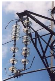
Figure 4. Insulators equipped with arcing horn and damages due to back flash over or shielding failures on 150 kV lines
