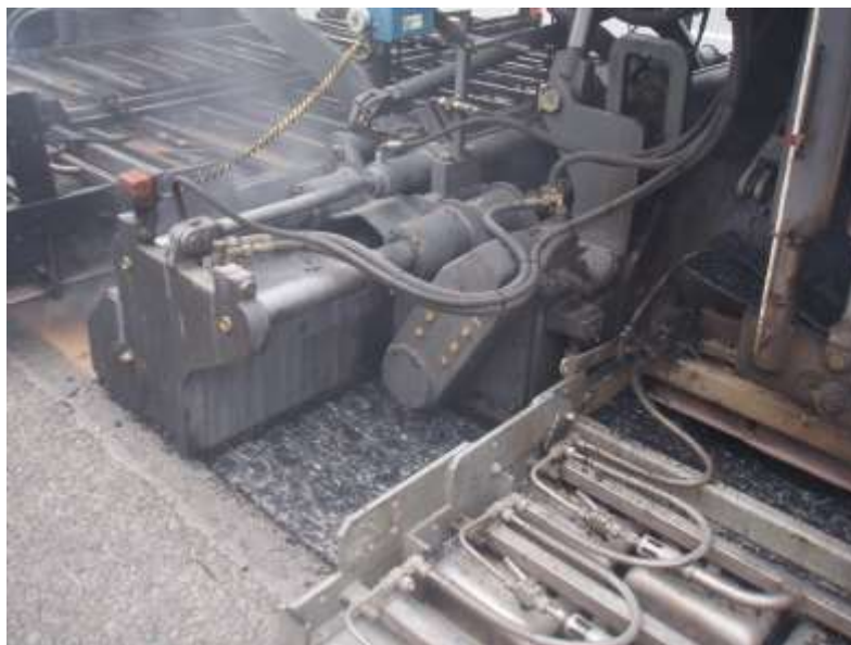
Figure 6. Scarifying and heating unit
