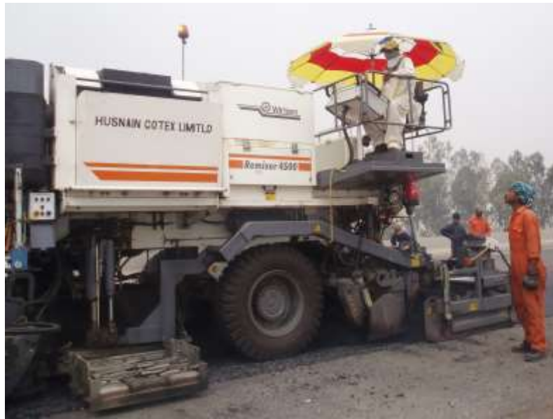
Figure 7. Remixing unit
