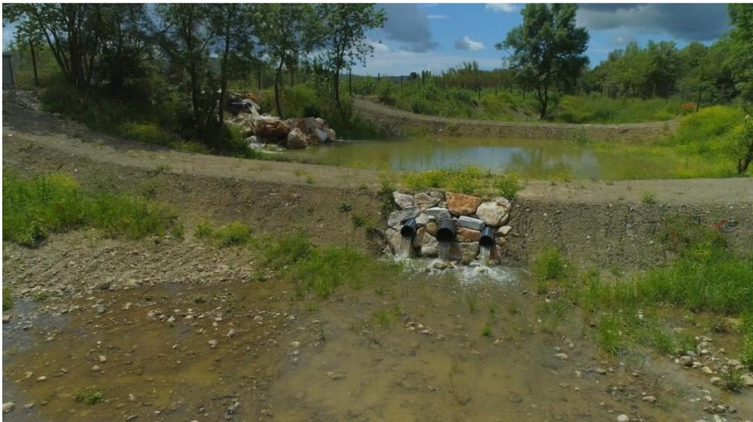
*Fig. 1 - View of the inlet point and detention basin, and discharge into the infiltration basin*
