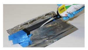
Using a mat and gloves, carefully fill U profile with construction foam. Let the foam extend into all cavities, and make sure there are no bubbles. Let foam set according to instructions (or overnight).
