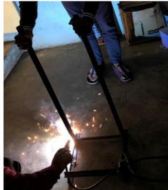
**Fig : 13.** Welding Of Supporting Columns
