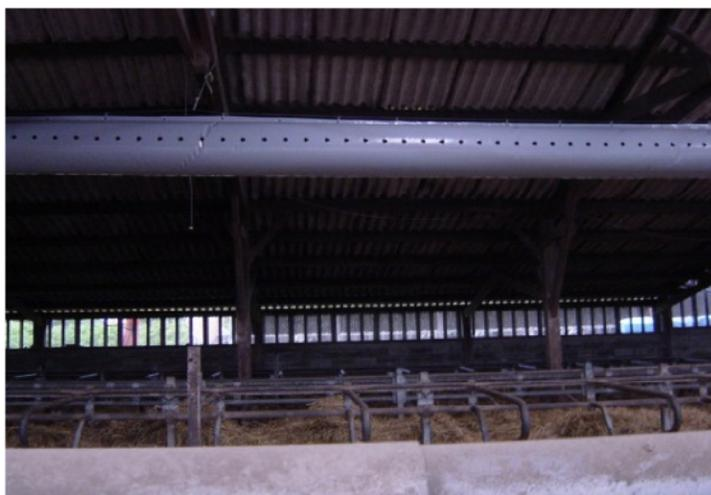
**Figure 7.** Duct for dispersing an artificial tracer gas within an animal house.
