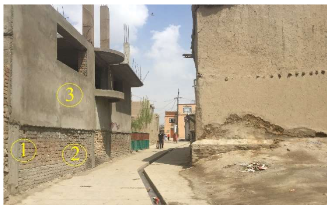
Fig. 5 A modern reinforced cement concrete (RCC) type house with the cement plaster used on the walls *1-RCC column, 2-Baked bricks wall, 3-Cement plaster
